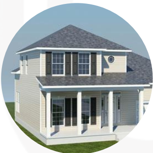
Hip Roof, Moderate Pitch
